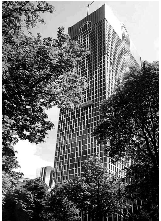
The Frankfurt office of Mannheimer Swartling has recently moved into this office building at Bockenheimer Landstraße.
